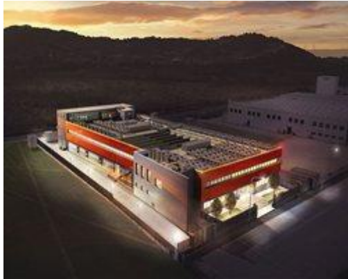
Figure 1 – Data Center IT1
