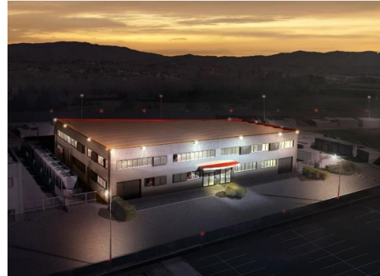
Figure 2 – Data Center IT2
