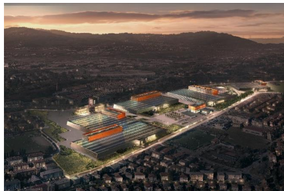
Figure 3 – Data Center IT3
